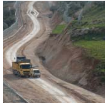
Construction of the Separation Barrier in Jerusalem. Photo: B'Tselem
