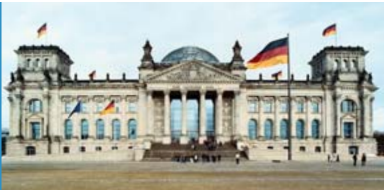
Reichstag Building viewed from the west.
