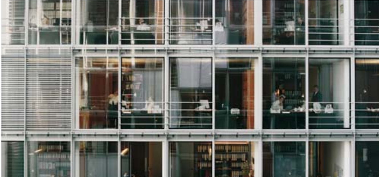
Each office measures 19.2 square metres.
